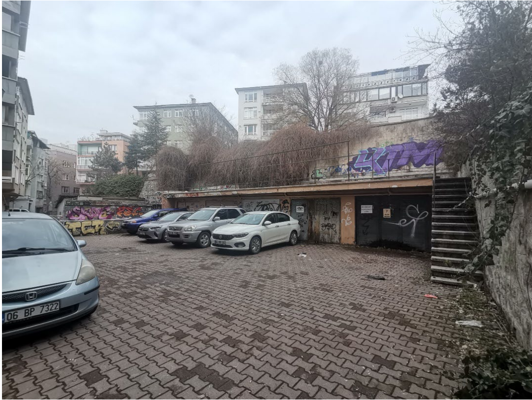
Figure 37. Illegally built closed parking garage.
